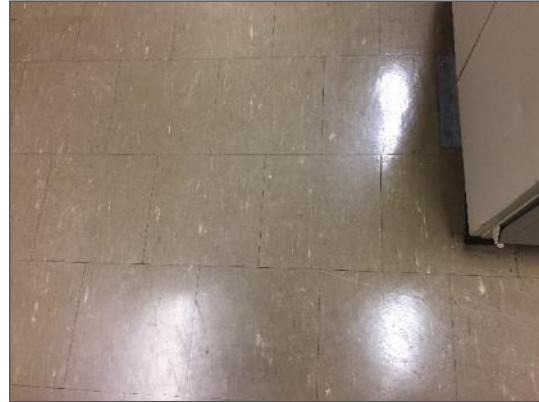
Asbestos-containing 12" x 12" vinyl floor tiles, brown with white flecks.
