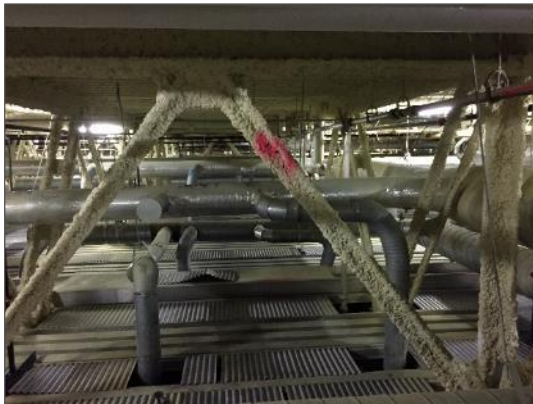
Encapsulated asbestos-containing sprayed fireproofing on structural steel, Level 2M Interstitial.
