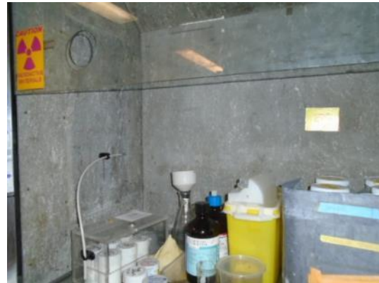
Transite board in typical fume hood, Level 4 Laboratory.
