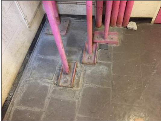
Asbestos-containing 12" x 12" vinyl floor tiles, dark brown with brown flecks.
