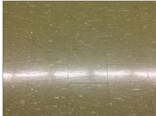
Asbestos-containing 12" x 12" vinyl floor tiles, green with white flecks.
