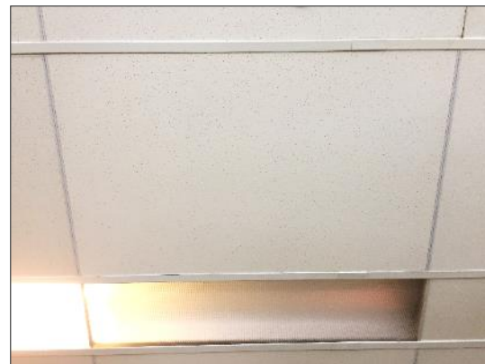
Non-asbestos lay-in ceiling tiles, uniform pinhole pattern, Level 4 Stairwell 56.
