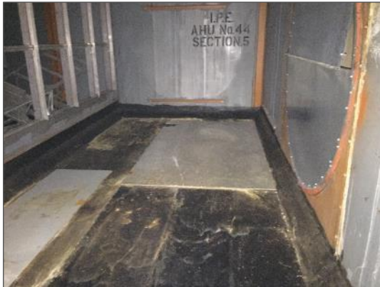
Transite board in air handling unit, Level 6 Mechanical Penthouse.
